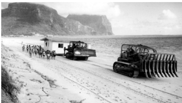
Jean Brierley's house is relocated – 29 March '74.
