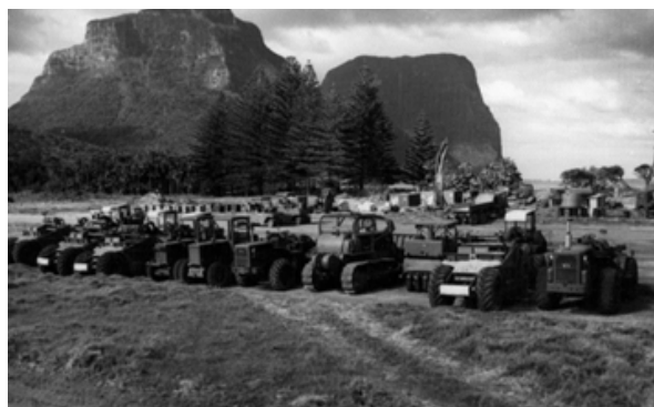
Machinery used to form the airstrip.
