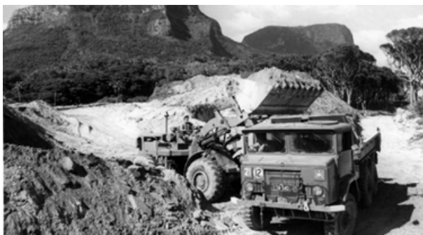
Excavation of Kirribilli Hill to provide pavement material for the airstrip – from late March, '74.
