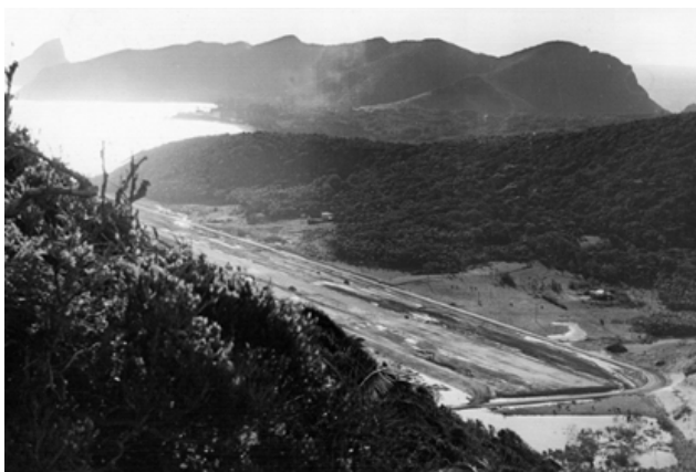
Progress on the airstrip – May, '74.
