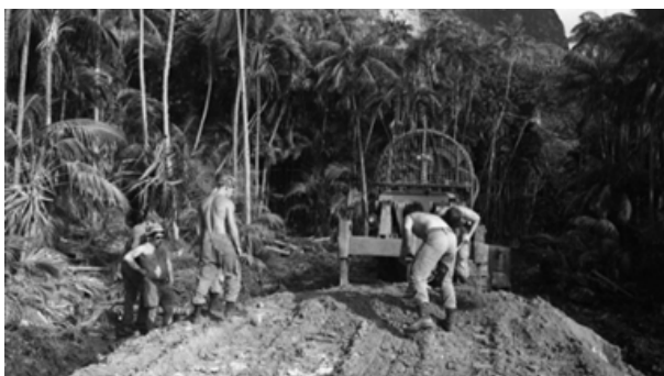
After the road to Little Island is constructed, rocks were trucked from the boulder beach there to the lagoon end of the airstrip, where they formed a protective sea wall against tide and wave.
