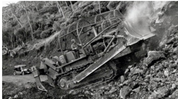
Jamie Elliot on D-8 bulldozer - Little Island Rd.
