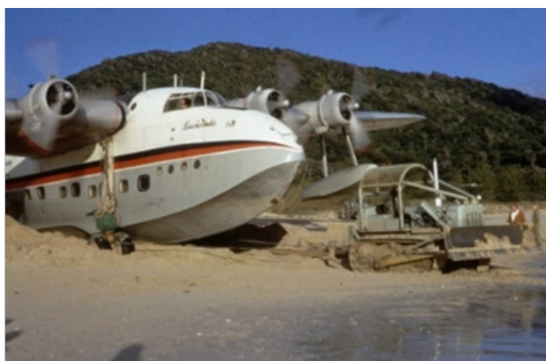
A dozer pulls whilst the aircraft engines are gunned.
